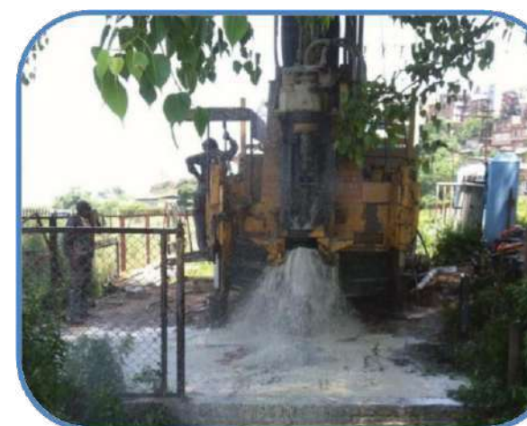
Deep Tubewell Drilling Work
