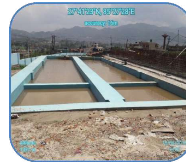
Sedimentation Tank Rehabilitation at Bansbari Bhaktapur
