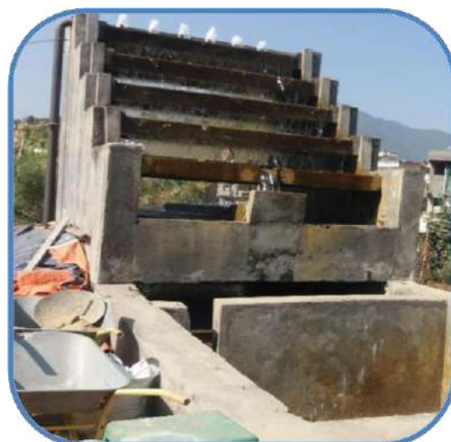
Cascade Aeration (Before and After)
