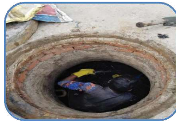
Removal of Sludge and Jetting Activity
