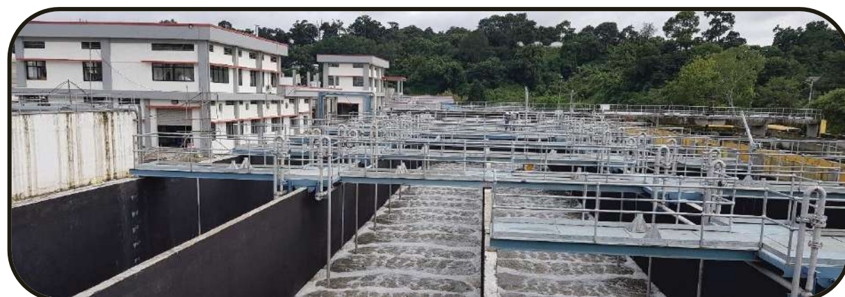
Guheshwori Treatment Plant (Aeration Tank)
