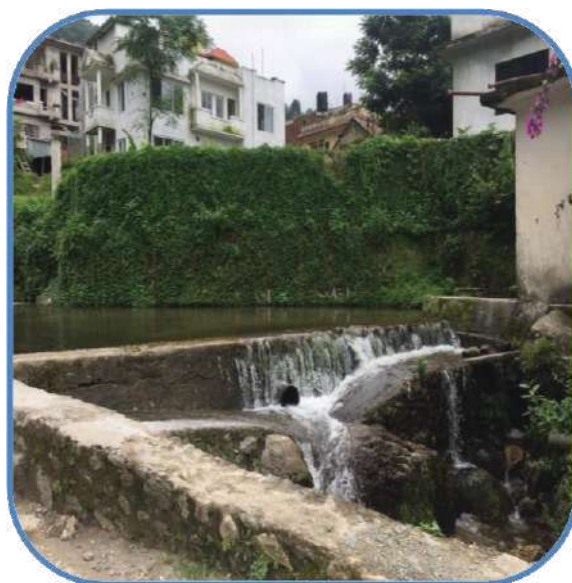
Old Intake Structure
