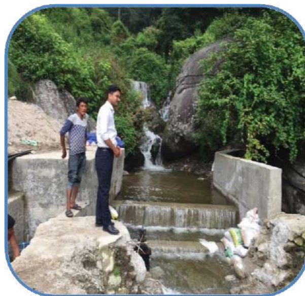
New Intake Structure
