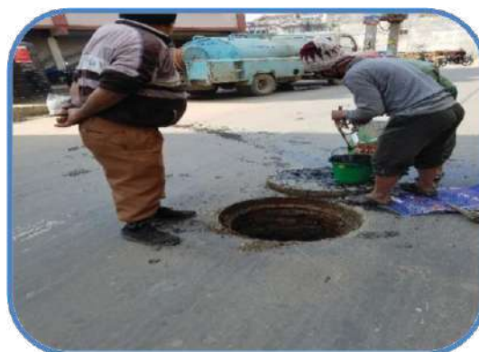
Removal of Sludge and Jetting Activity
