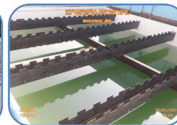
Sedimentation/Clarifier at Sundarijal
