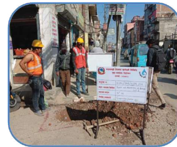
Leak Repair Works by PMU
