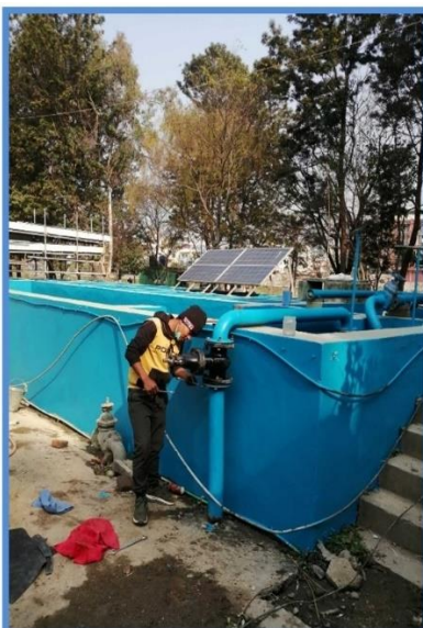
Rehabilitation of existing BPT at Shikhar Pa Lalitpur
