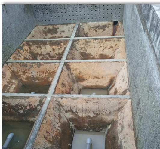
Sludge Removal Works from Sedimentation Tank
