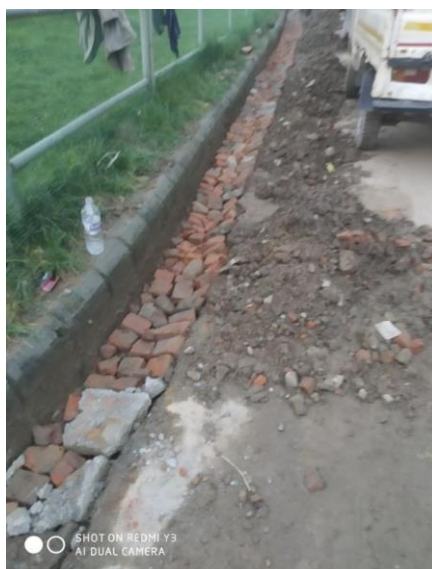
250 mm dia DI Transmission Main Protection Work at Nallu River Crossing
