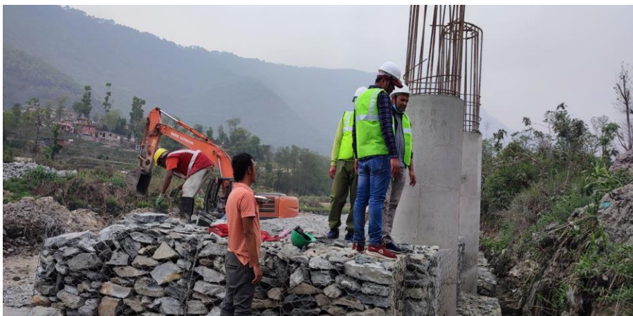
Construction of Truss Bridge for 400mm dia DI Transmission Main Crossing at Bagmati River, Khokana Lalitpur
