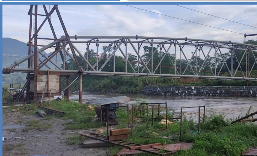
Construction of Truss Bridge for 400mm dia DI Transmission Main Crossing at Bagmati River, Khokana
