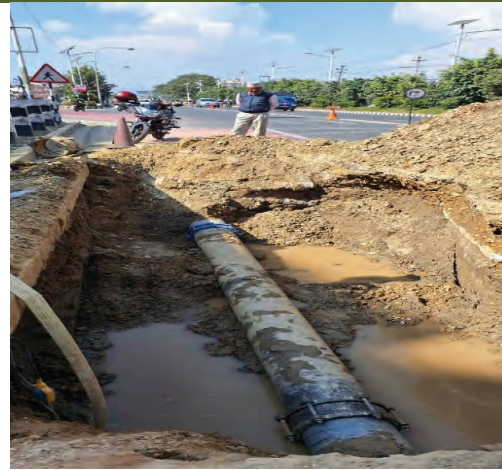
Leak Maintenance on 350mm dia UPVC Transmission Main at Tinkune
