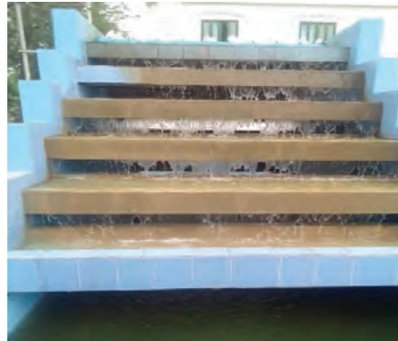
Aerator after installation of tiles
