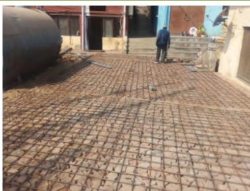
RCC Floor Construction at Sundari Ghat Water Treatment Plant
