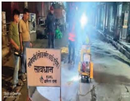
Pavement Cutting Work using Cutter for Replacement of 200mm dia CI Sluice Valve
