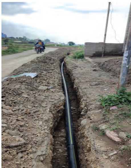
Laying and Jointing of 150mm dia HDPE transmission mains from Kirtipur SRT to Jhaka Tank
