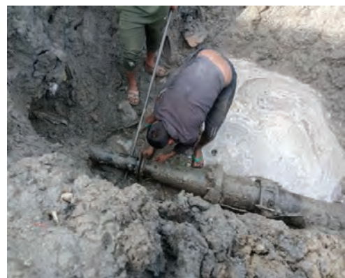
Leakage repair work in Baniyatar, Tokha-8 (200 mm pipe and 100 mm pipe connection)
