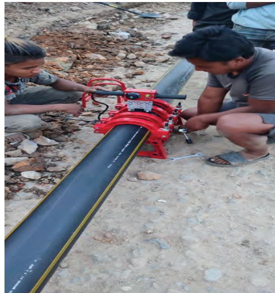
Butt Weld Jointing Work of 150mm dia HDPE transmission mains
