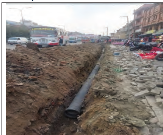
10" dia pipeline laying works at Jagati
