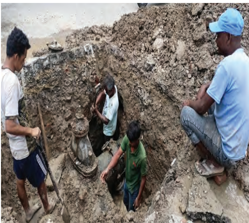
Leakage Repair work at Lainchaur in 400 mm pipeline
