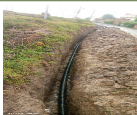
90 mm HDPE Pipeline Extension work at Shivnagar, KMC-14
