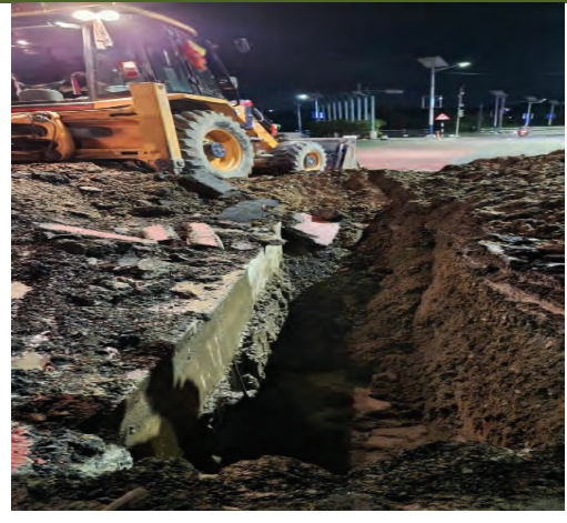
Leak Maintenance on 350mm dia UPVC Transmission Main at Tinkune
