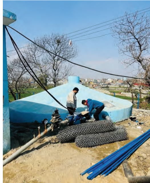
Semi-underground water tank of 115 cum.
