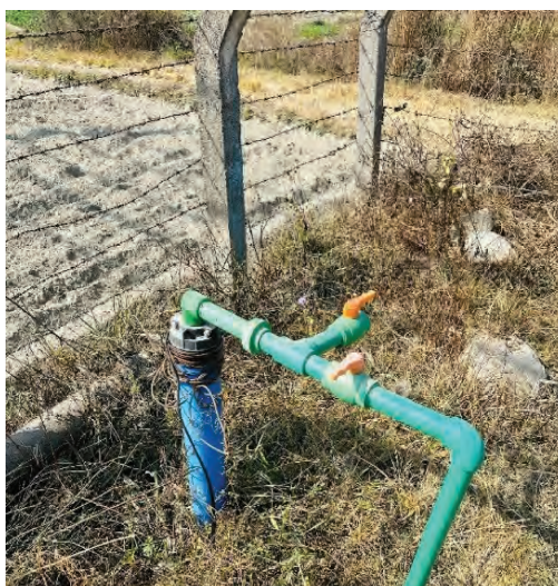
Addition of shallow wells at Manohara Dug wells.
