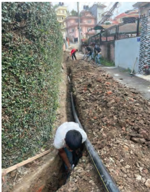
Pipeline extension work at Shreejanshil Marga
