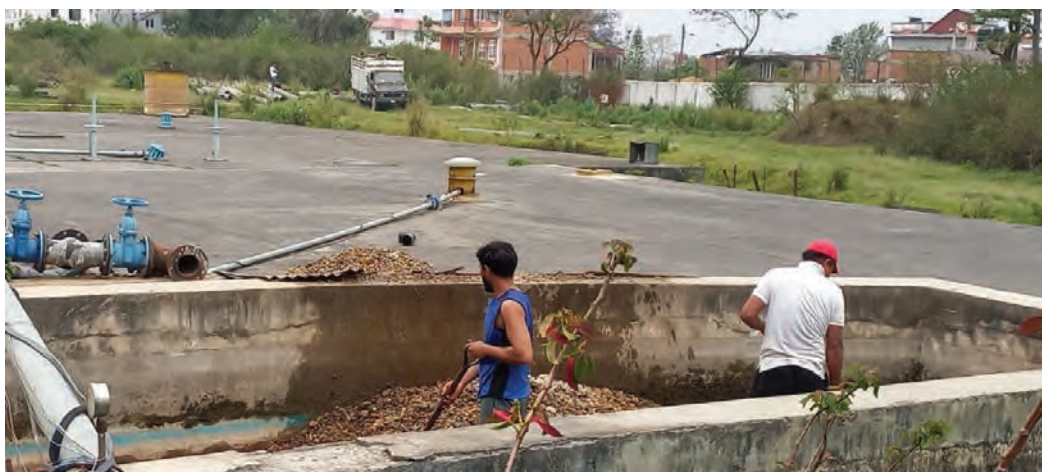
Replacement of filter media at Bhaisepti Water Treatment plant
