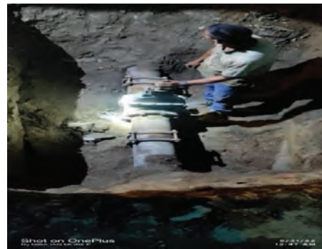
Replacement of 200mm dia CI Sluice Valve
