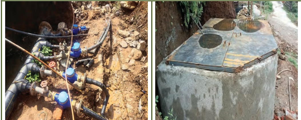
Installation of flowmeters and construction of flowmeter chamber
