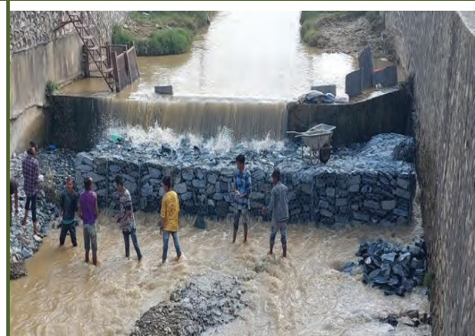
Gabion Wall Construction at Nakkhu Intake
