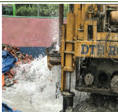
Drilling of new deep tubewell at Tarkeshwor Municipality-11, Kathmandu.
