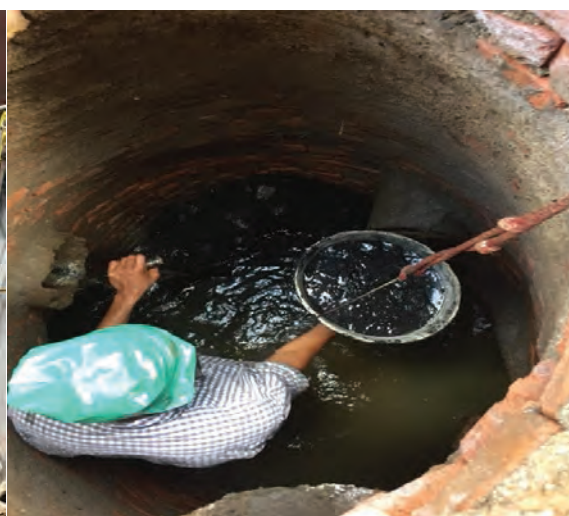
Cleaning of manhole at Buddhanagar area
