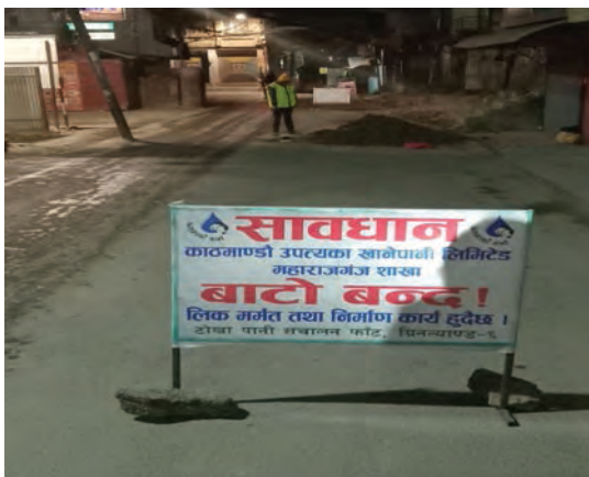
Safety work before commencement of repair work in pipeline
