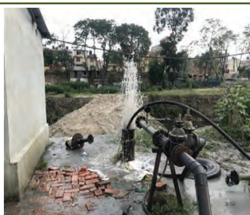
Well development by DTH (30 Bar) Compressor at Madhyapur Thimi, Gathaghar, Bhaktapur
