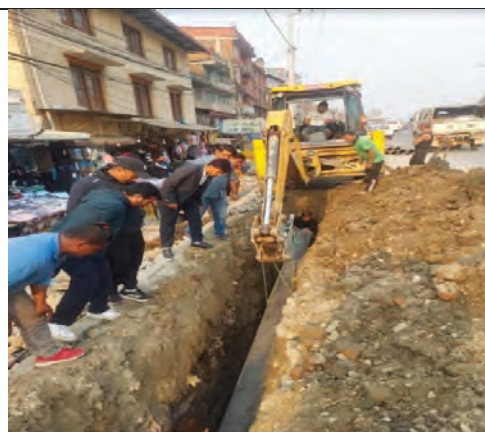
8" dia pipeline laying works at suryabinayak
