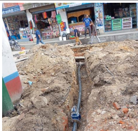
Pipeline interconnection (200mm x90mm) @ Radha Marg, Liverpool School Area etc. Baneshwor.
