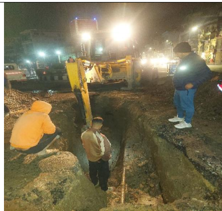
32" Dia CI Pipeline Repair at Chabahil chowk
