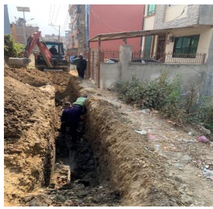
4" dia. pipeline improvement works at Kharibot area
