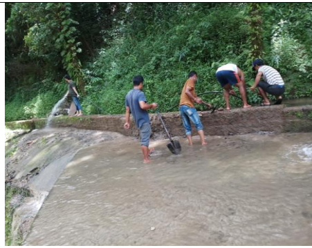
By-pass canal cleaning work at Mahadev Khola Muhan.
