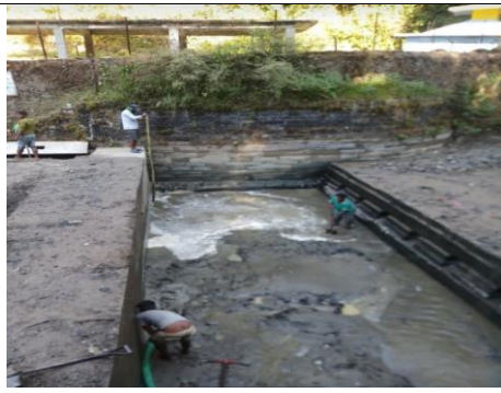
Mahadev Khola Muhan intake cleaning work.
