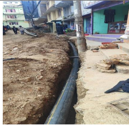
160mm dia. pipeline improvement work at Chiyan
