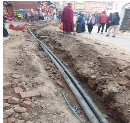
4" dia HDPE pipeline extension work at Baudha
