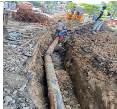
12" dia. Main pipe Relocation Work at Chauni hospital premises.
