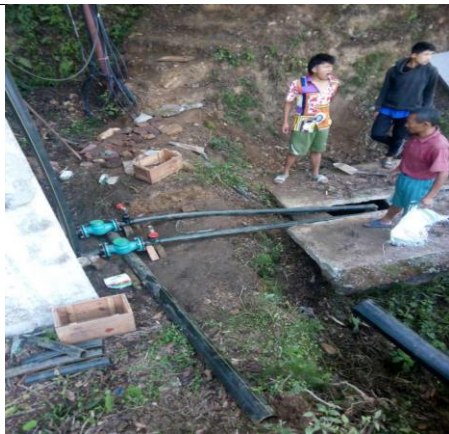
Installation of 50mm dia. Bulkmeter at Dudhpokhari
