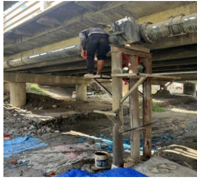
Maintenance of 14" dia. sluice valve at Lokanthali
