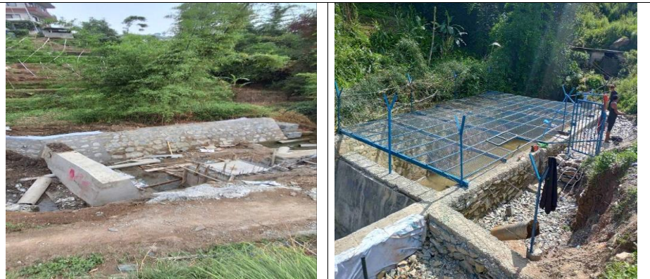
Construction of Check dam at Kutule Source at Pharping.
