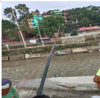
Pipeline protection work at KMC-19, during flood.
