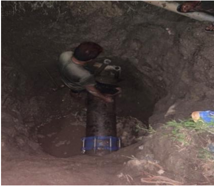
Plugging of 14" dia. transmission line at Manohara river
