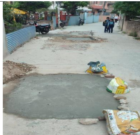
Restatement of road through RCC after leak maintenance work @ Ajima Park.
