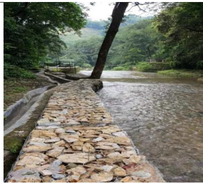
Gabion wall construction work at Mahadev khola Muhan.
