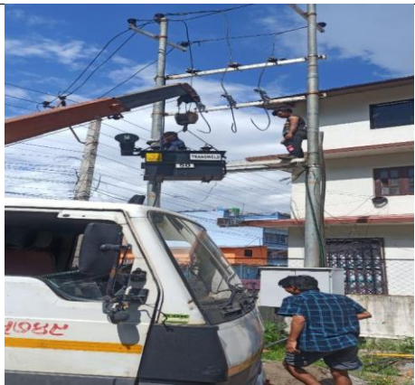
Installation of new transformer at Tarkeshwor-11 well, Kathmandu
