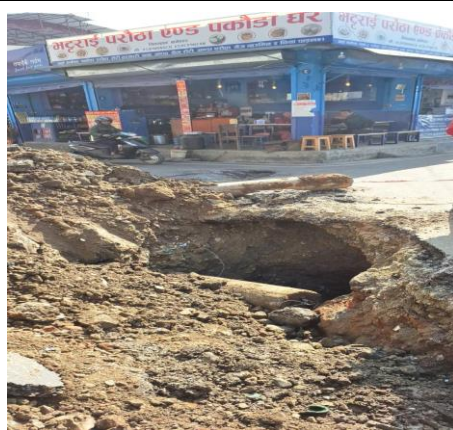
Leakage maintenance works @ Nepal Commerce Campus Minbhawan, Baneshwor.
