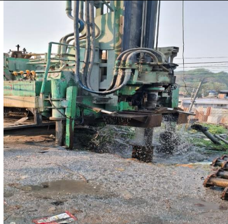
Drilling of new DTW @ Kamaretar, Thimi,
