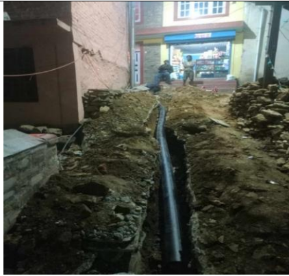
160mm dia. Pipeline improvement Work at Chovar
