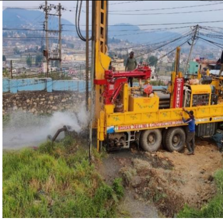
Well development by DTH (30 Bar) Compressor at Basbari tube well, Bhaktapur
