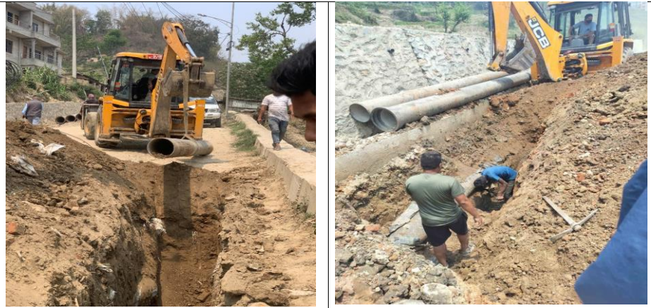
350 mm dia DI Pipeline extension work at LMC-22, Pharsidol to Bungmati.
