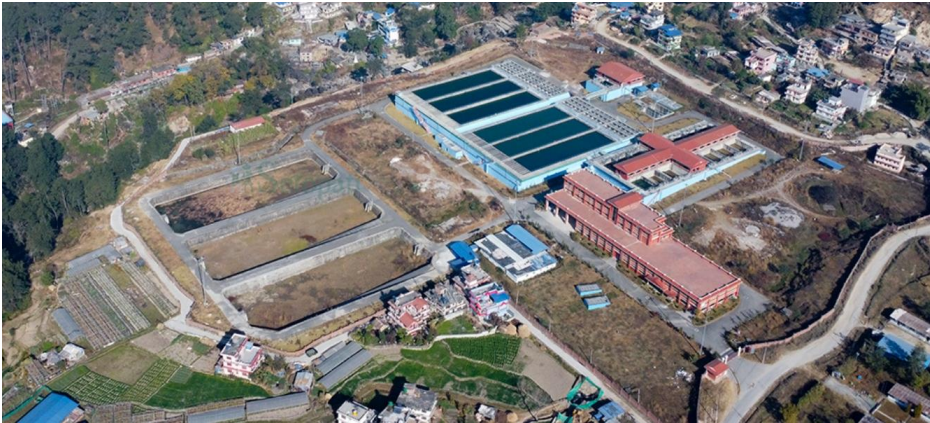
Sundarijal Water Treatment Plant
