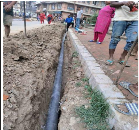
4" dia. HDPE Pipeline laying @ Gokarna shivapuri Area
