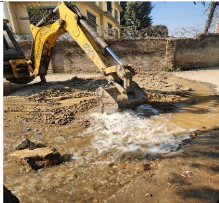
16" dia CI Pipeline Repair works at Mulpani area
