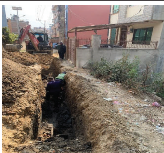
4" dia. pipeline improvement works at Kharibot area
