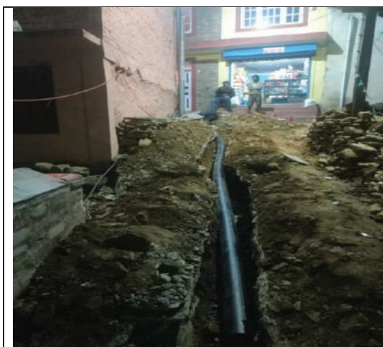
160mm dia. Pipeline improvement Work at Chovar
