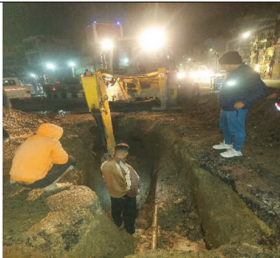
32" Dia CI Pipeline Repair at Chabahil chowk
