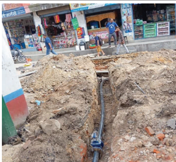
Pipeline interconnection (200mm x90mm) @ Radha Marg, Liverpool School Area etc. Baneshwor.
