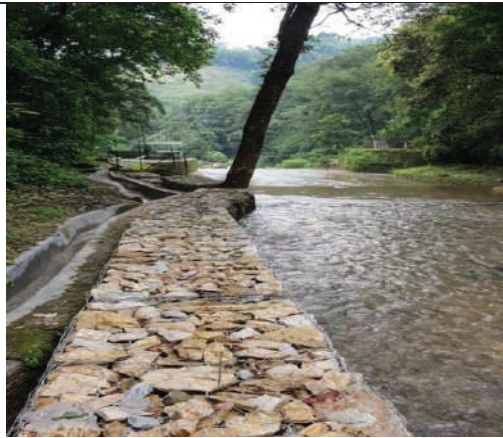
Gabion wall construction work at Mahadev khola Muhan.
