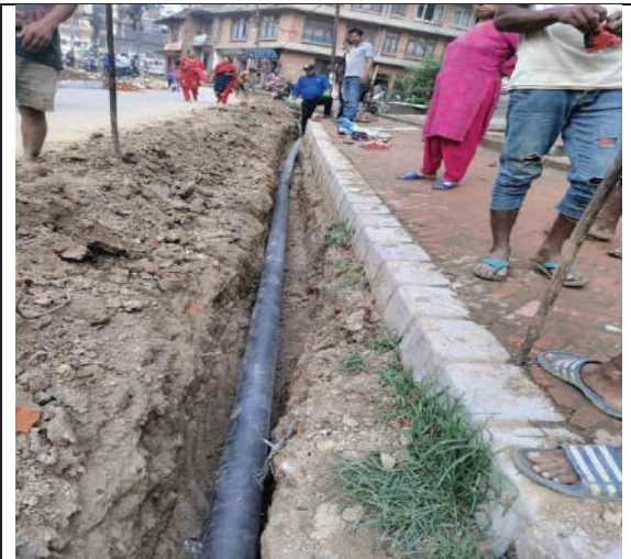
4" dia. HDPE Pipeline laying @ Gokarna shivapuri Area
