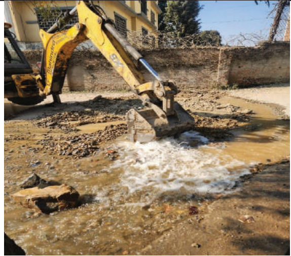
16" dia CI Pipeline Repair works at Mulpani area
