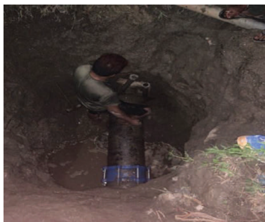
Plugging of 14" dia. transmission line at Manohara river
