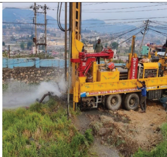
Well development by DTH (30 Bar) Compressor at Basbari tube well, Bhaktapur
