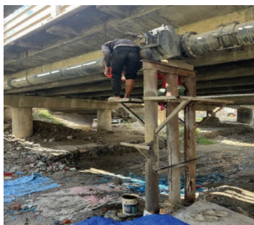
Maintenance of 14" dia. sluice valve at Lokanthali
