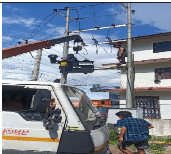
Installation of new transformer at Tarkeshwor-11 well, Kathmandu
