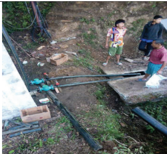
Installation of 50mm dia. Bulkmeter at Dudhpokhari
