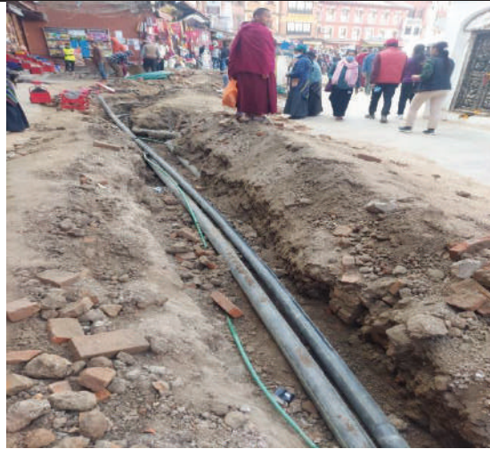
4" dia HDPE pipeline extension work at Baudha
