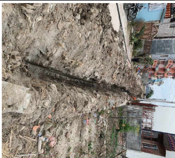
4" dia. pipeline extension work at Gankhu
