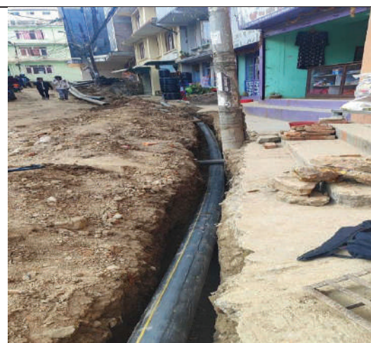
160mm dia. pipeline improvement work at Chiyan
